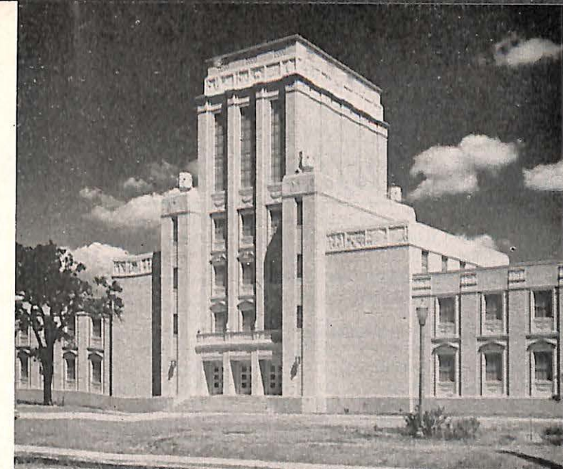
The new, five-story Tidwell Bible Building on Baylor University Campus, Waco, Texas, where some of the North American Baptist General Conference meetings will be held
