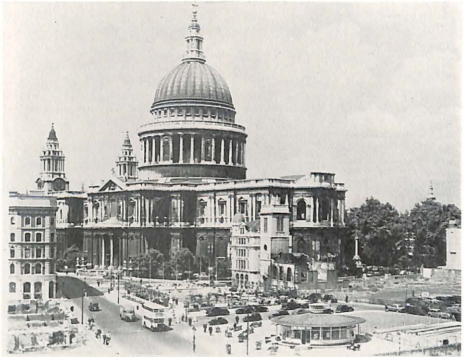
St. Paul's Cathedral in London, England, which was built after the Great Fire of 1666 by Wren on the site of Old St. Paul's. Work was completed in 1710
