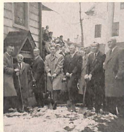
Ground breaking exercises for the $20,000 addition to the Second Baptist Church, Union City, N. J., with church leaders and Rev. R. Sparling, pastor, taking part.
