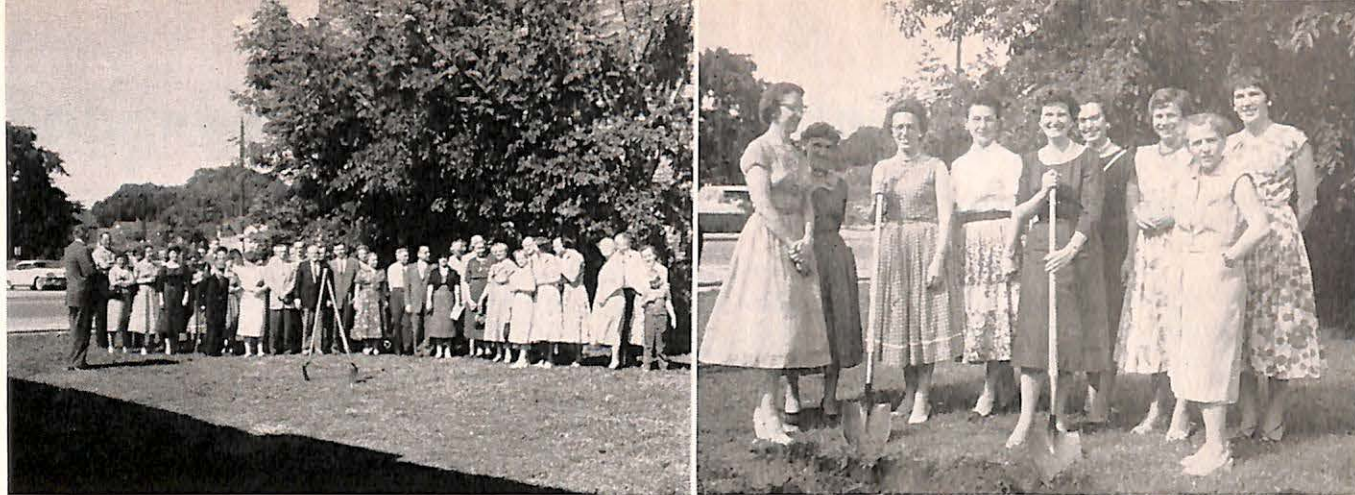
GROUND IS BROKEN FOR NEW BUILDING IN FOREST PARK
