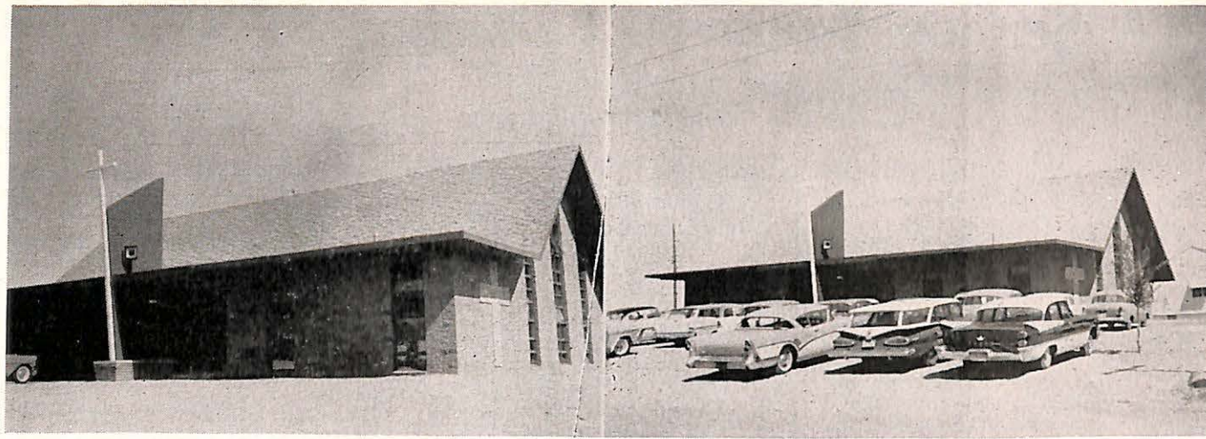
THE $100,000 NEW BAPTIST CHURCH IN PLEVNA, MONTANA
