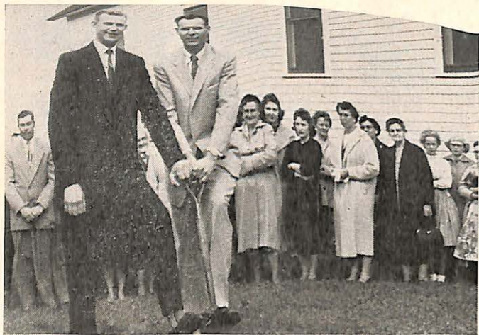
Ground is broken for the new addition to the Jeffers Baptist Church, Jeffers, Minn., with Duane Carlblom (left, foreground) and Rev. David J. Miller, pastor, at the right (holding shovel).
