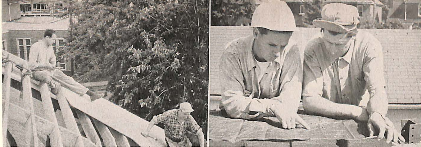
NEW CHURCH UNDER CONSTRUCTION, HAMILTON, ONT.
