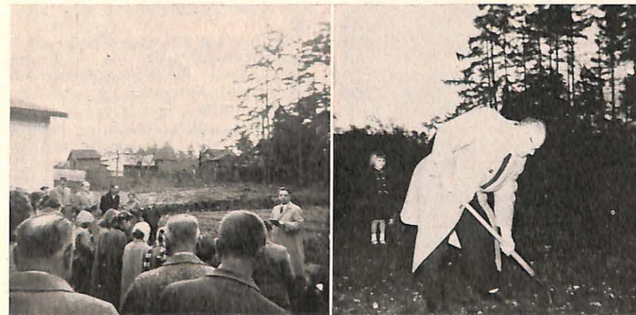
GROUND BREAKING EXERCISES AT TACOMA
